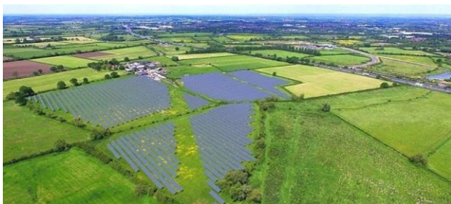
Swindon Common Farm Solar
